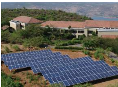
Ground Mounting Project
